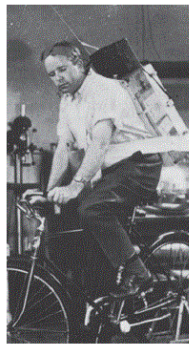
Figure. Jeff Hottel with his original 38-kg radio-electronic and logograph recording device in 1947.
